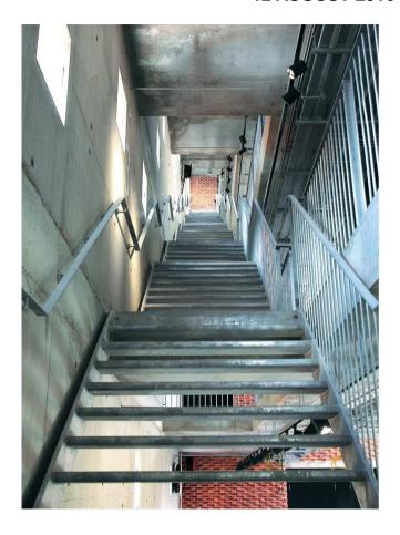
One of the distinctive traits of the centre is the straight-flight steel staircase. The visually transparent-looking stairs create crossventilation and a sense of flow and unification of all the floors and spaces in the building.
