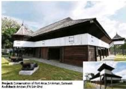
Project: Conservation of Fort Alice, Sri Aman, Sarawak Architect: Arkitek JFN Sdn Bhd
